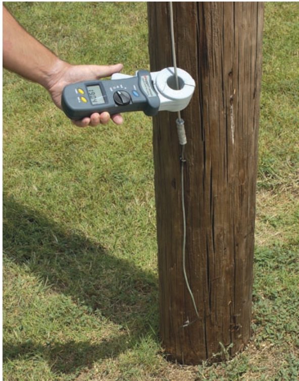
The DET20C instrument is shown being used to test a pole ground.
