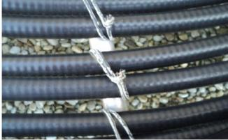
Figure 5. Improper Cable Camps
