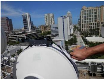
Pull excess webbing strap so that it is snug on the antenna.
