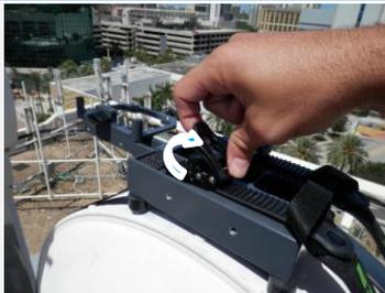
Ratchet the ladder strap through the buckle until webbing is tight on the antenna. Repeat steps for second webbing strap to secure the clamp.
