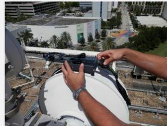
Insert ladder strap into the ratchet buckle just enough to engage, approximately 1".
