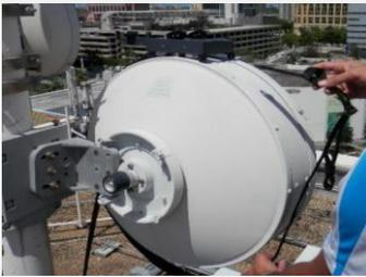
Position strap clamp body with rubber bumpers on the drum antenna. Wrap webbing strap around antenna.
